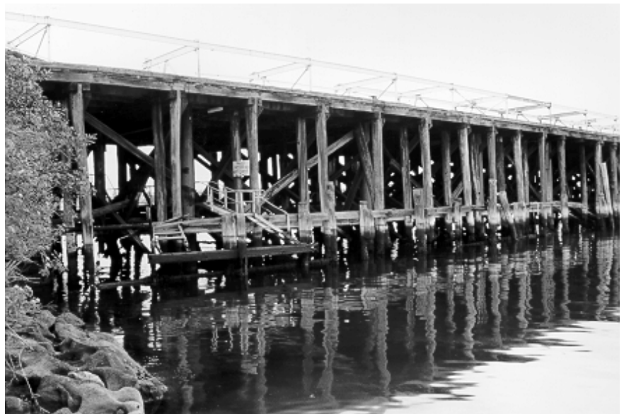
Figure 6.27 High level timber industrial wharf, reinforced with steel in 1976.
