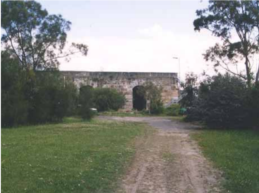
Figure 3.4 The Coal Loader platform and tunnels are major landscape elements.
