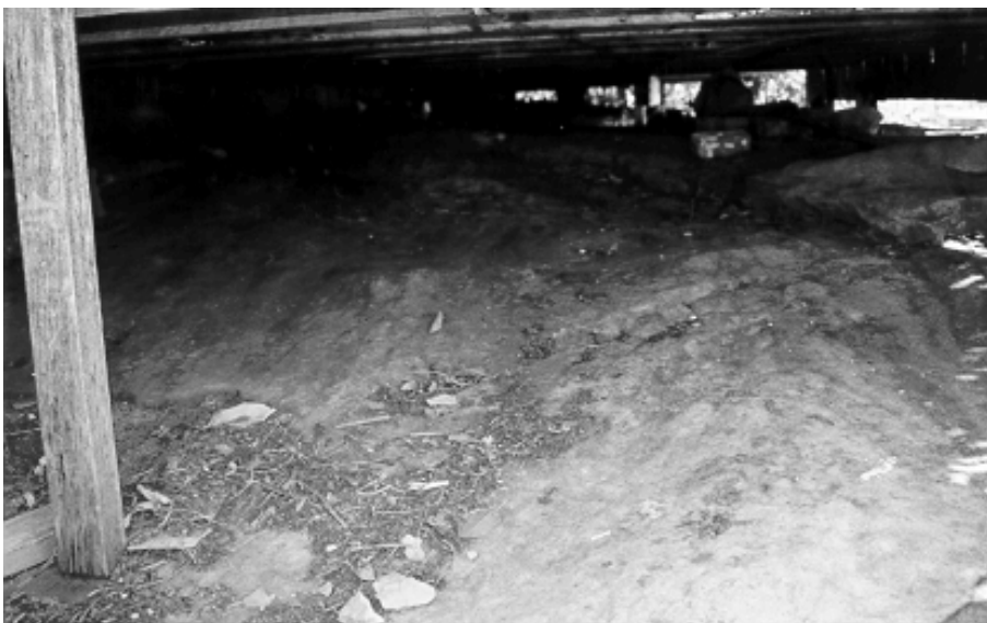
Figure 4.20 Sandstone surfaces below timber patio of Coal Loader residence.
