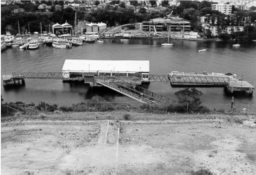
Figure 6.12 1962 concrete Dolphin wharf connected by steel walkways. Note 1926 lower terrace in foreground.
