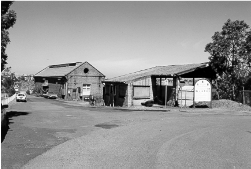
Figure 13.9 Entry to Coal Loader site from Balls Head Road with access to HMAS Watershed on right. Building left of centre is former Fitters' Workshop and Powerhouse, now converted to offices by lessee.
