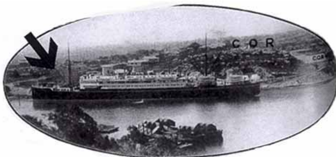
Figure 5.6 The COR. installation at Berrys Bay in 1933, with the MV Wanganella loading diesel in the foreground. Of interest in this photograph is the still standing stone store just behind the foremast of the vessel ('The Accelerator', 18 February 1933).
