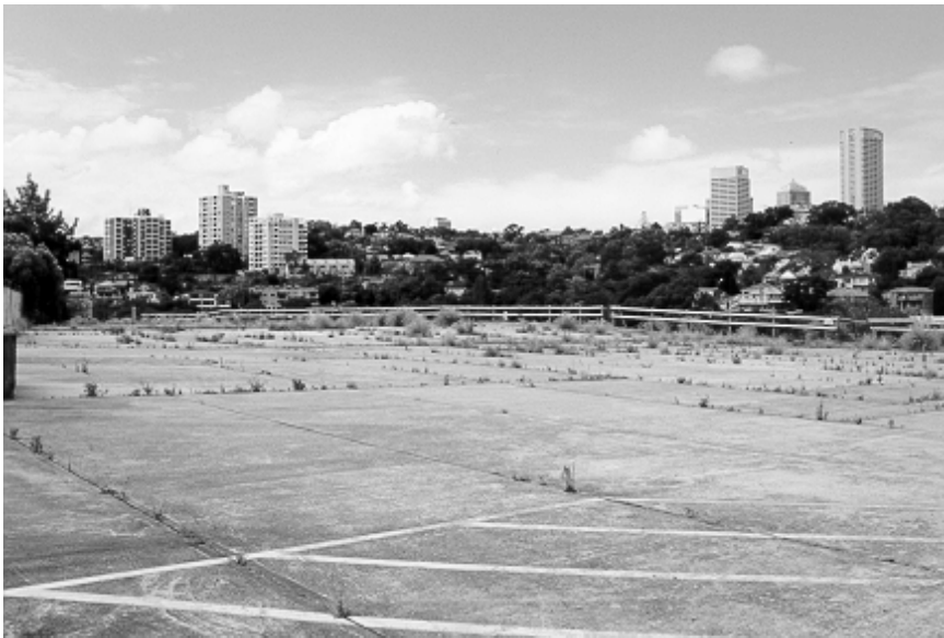
Figure 6.4 The c1960s concrete retaining wall was built to form a flat area for road fuel tankers at the Larkin Street level. The upper wall and lower excavated rock and 1926 terrace in the foreground are features of this modified distinctive industrial landscape.
