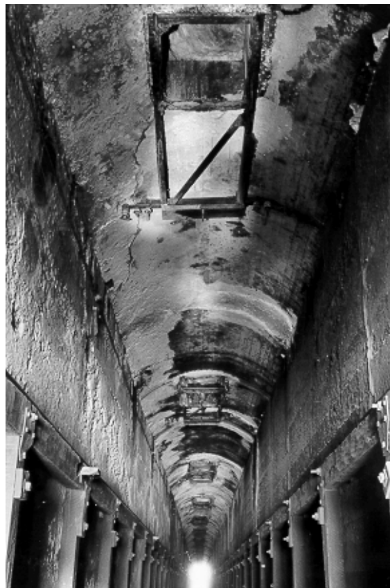
Figure 6.23 Original bin gates in tunnel No. 1 from the base of the hoppers in the Coal Loader platform.
