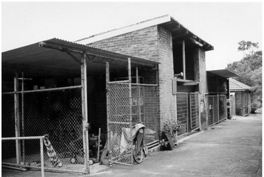
Figure 6.35 Welding shop/blacksmith's/ carpenter's workshop and WC. The central high section and steel-framed open area in foreground are original.
