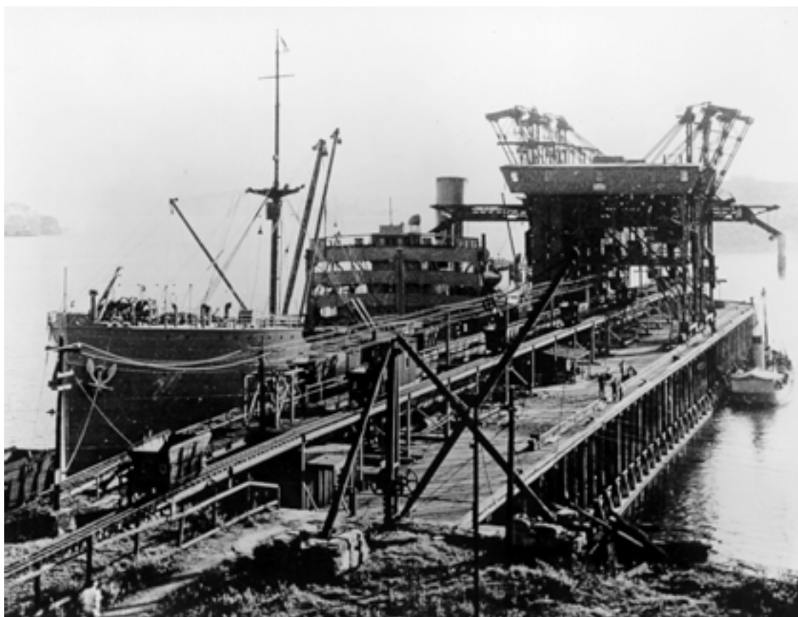
Figure 5.15 SS Port Cardine being charged with coal at the Balls Head Bay facility, 3 May 1940. The wagons are clearly seen running along the railway to the loader (Stanton Library, PF1165).
