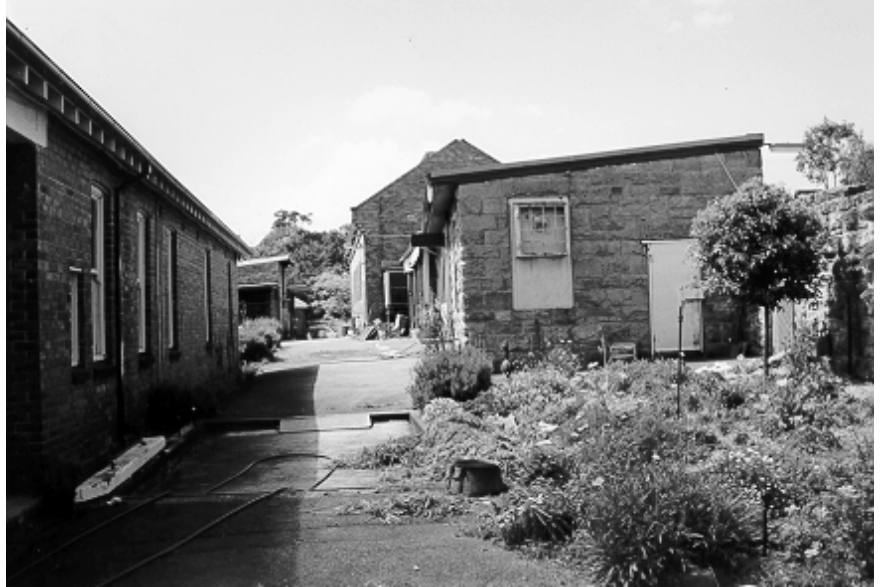
Figure 6.34 Original sandstone site office, RHS, and brick administration building, built soon after with weighbridge between. The powerhouse and workshop/forge are in the background.
