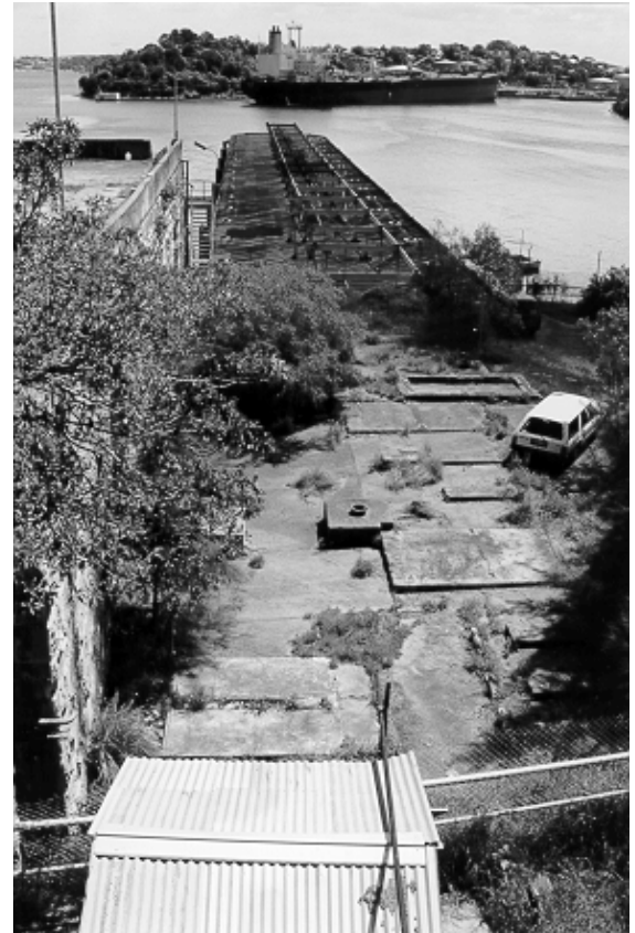
Figure 6.30 View from Balls Head Road level, along the northern side of the coal platform, and wharf. Note the concrete foundations of 1976 conveyor structure and equipment. The original timber stairs connecting the two levels extended from the base of the photo.
