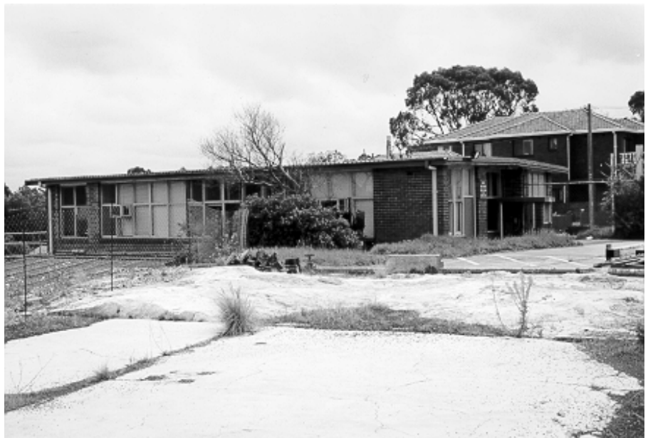
Figure 6.3 1960s brick office for BP at Larkin Street. The foreground shows the potential archaeological site as a pre-1923 store room.
