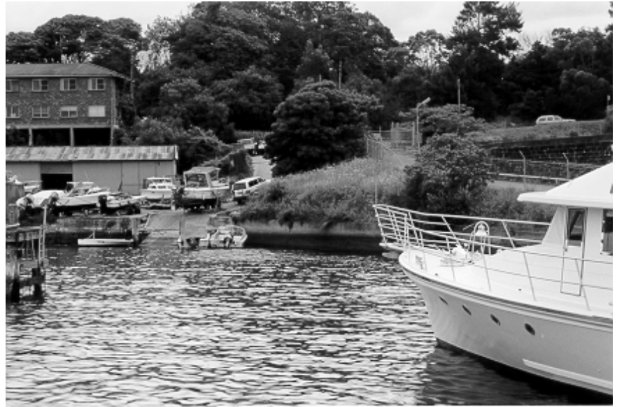
Figure 6.6 Woodley's Boat Yard, Berry-era boat ramp and sea wall, and overgrown sandstone block wall above concrete sea wall, in vicinity of Berry's sandstone quay-style wharf.
