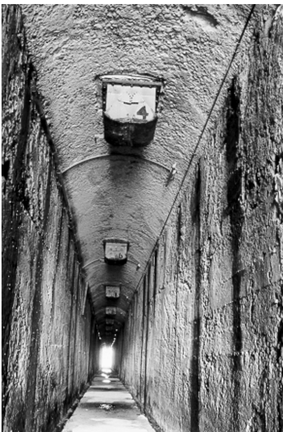
Figure 6.25 1976 geared bin gates in situ in tunnel No. 2. The numbers correspond to the hopper number above.
