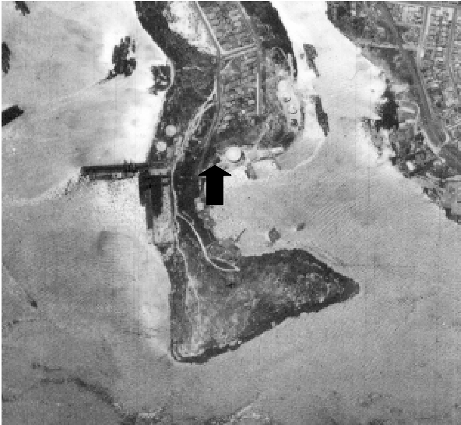
Figure 5.16 Aerial photograph of the BP and Coal Loader site c1935. On the BP site Berry's store is just visible next to the main storage tank. Two storage tanks are also visible to the north of the Coal Loader.
