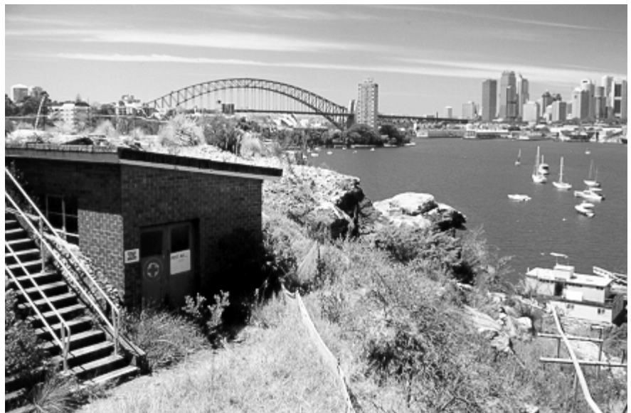
Figure 13.8 View from BP office to city and Bridge showing First Aid Hut which can be demolished.
