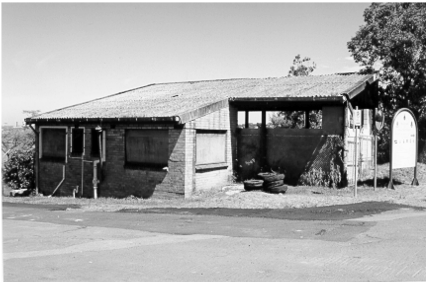
Figure 13.10 Coal Loader site. Former Mess Room could be adapted as short or long-term Visitor Centre. It is conveniently located at northern end of site, closest to public transport and is close to the Aboriginal rock art site. Corrugated asbestos cement roof would need replacing.
