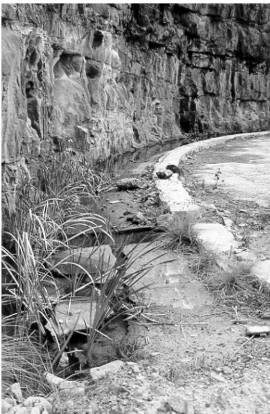
Figure 6.9 The removal of the steel fuel tanks in 1994 revealed the dramatic excavated sandstone walls, canals and concrete bases for the tanks.
